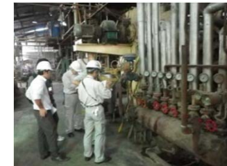
A Yokohama company at work on site
