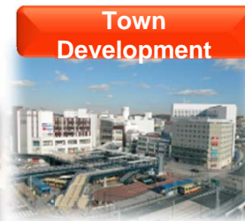
Re-development of the West Gate of Totsuka Station
