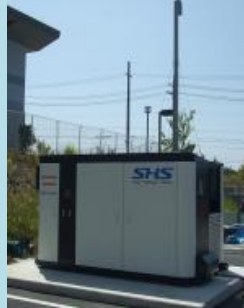
Kobe renewable energy hydrogen station
