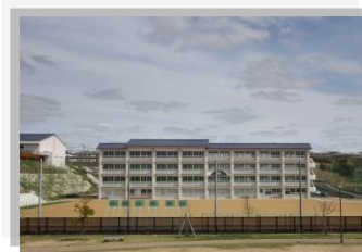
The exterior of Maitamon elementary school
